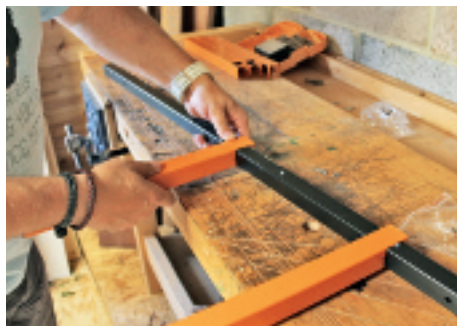
▲ Each support is slid into place and the next screw inserted
