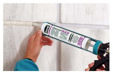
For joints subject to high casting or setting out tolerances the joint depth should be a minimum of 10mm. For accurately formed joints in glass or metal the minimum depth can be reduced to 6mm.
