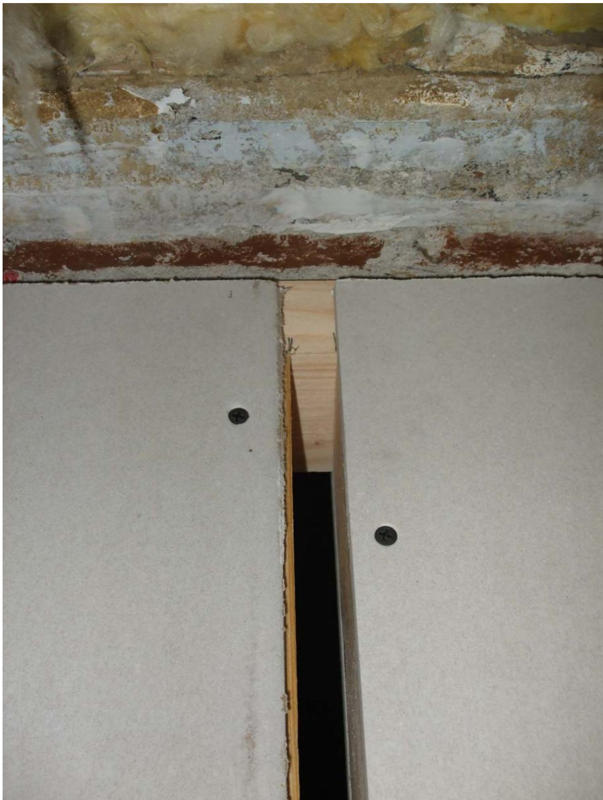
**Photograph 3: Fully Sealed Partition Close-Up**
