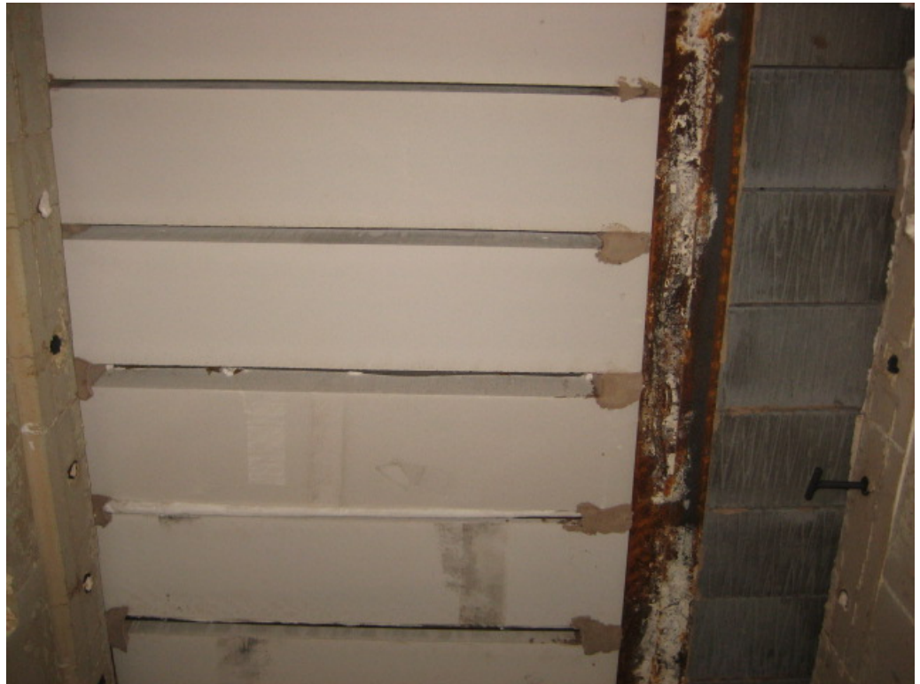
The exposed face of the floor construction prior to testing
