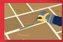
Finish the surface decoratively giving a smooth, flat finish with a pointing tool then move onto the next area. Firm compaction is the key to the successful laying of Geo-Fix All Weather Jointing Compound.
