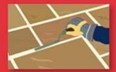
Firmly compact the Geo-Fix All Weather Jointing Compound with a pointing tool, refill and repeat ensuring a fully compacted and topped up joint.
