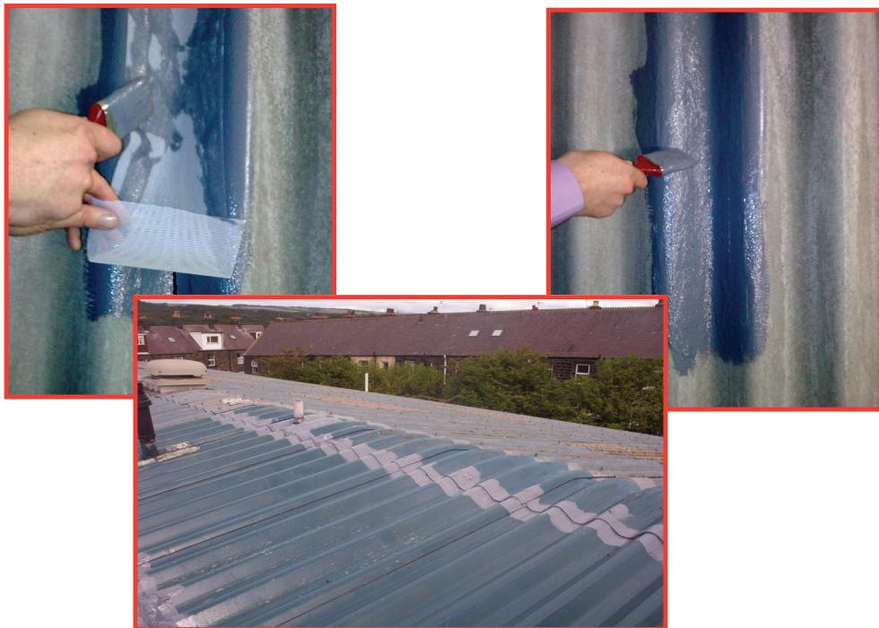
The product is thin enough to be absorbed into a single application of **ACRYPOL+** which means there are no visible seams or laps showing. The product has a unique rigidity which means it does not curl up on its edges in the way that some other products do. The more recent legislation relating to the use of heating equipment on roofs make this cold applied system a firm favorite with specifiers and contractors alike.
